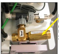
Pressure Regulator (Permeate Flow Control) Adjust with Blend Valve Closed
