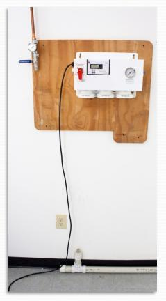
Step 2 Attach Water Processor at the upper and lower keyhole mounts.
