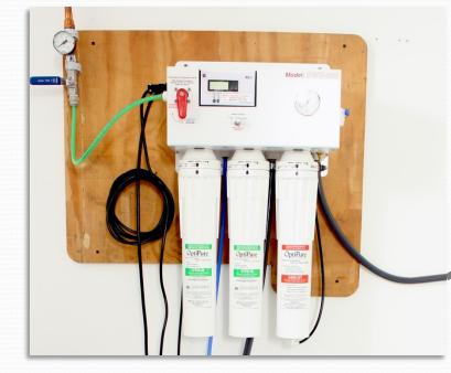
Step 16 Connect Optimized Water Line to Post-Treatment and downstream equipment.
