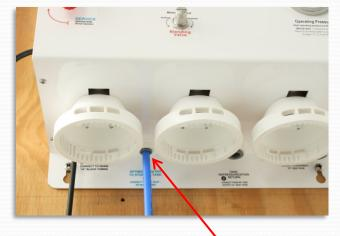
**Step 5a** Connect 3/8" Blue Tubing to "B" Optimized Water To Storage Tank.
