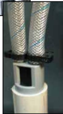
R. Drain hoses connected to air gap at drain pipe
